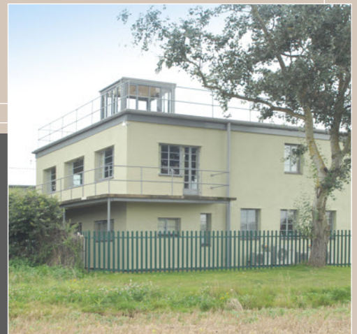
Photo of Award Winning refurbished Old Control Tower at Rackheath.
